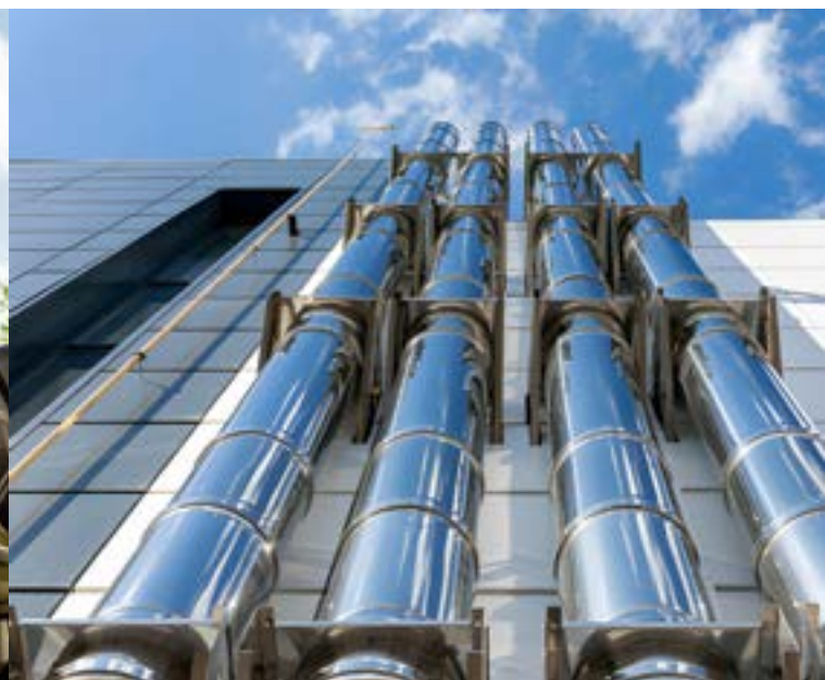
CHW Piping, Insulation and Cladding
